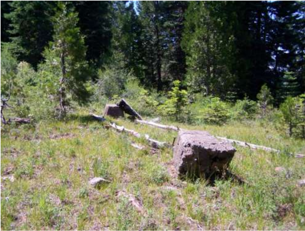
A few remnants of the foundation is all that remains of a fire lookout that once topped the now generally tree-obstructed view at the top of Anderson Mountain.
